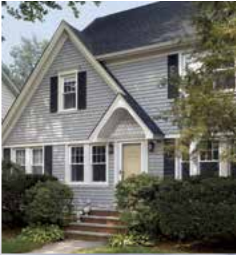
Siding: Triple 5" Straight Edge Perfection Shingles in sterling gray and Half-Rounds in colonial white. Trim: Vinyl Carpentry® & Restoration Millwork®.
